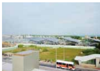
⬆ Magong Airport - BIPV (Building- integrated photovoltaic) demonstration project.
