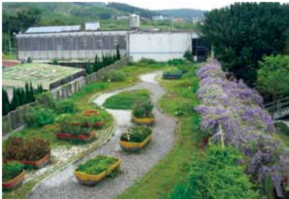
The school's green roof and solar power electricity generating installations.
